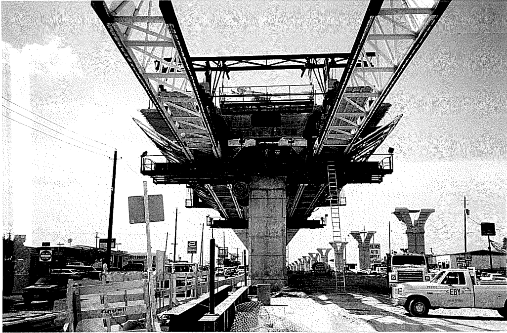
Figure 4.6 - Pier Bracket Supporting Truss
