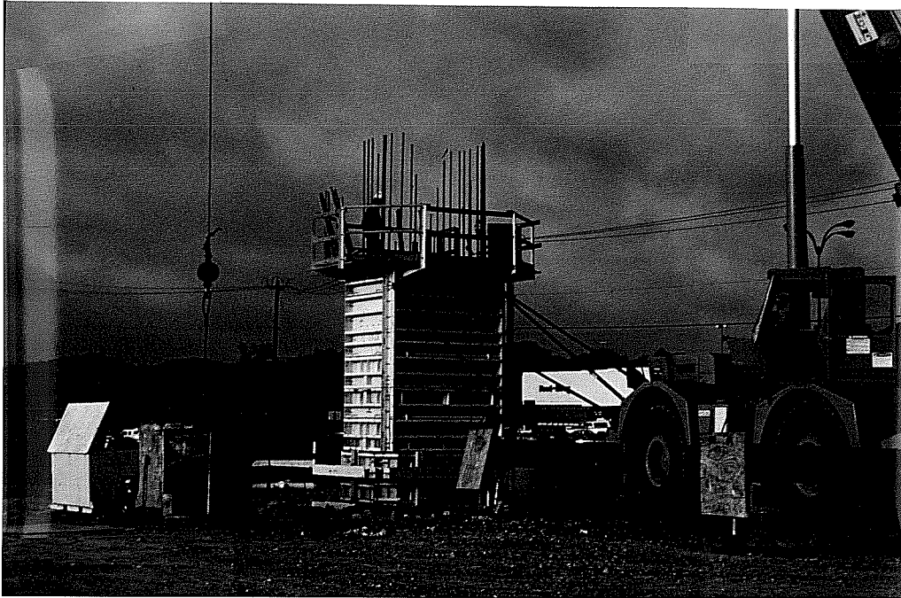
Figure 4.1 - Casting of Pier Column Concrete
