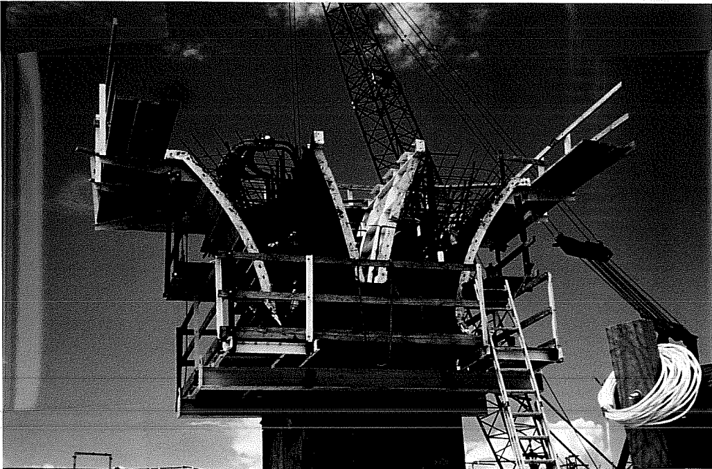
Figure 4.2 - Construction of Pier Capital
