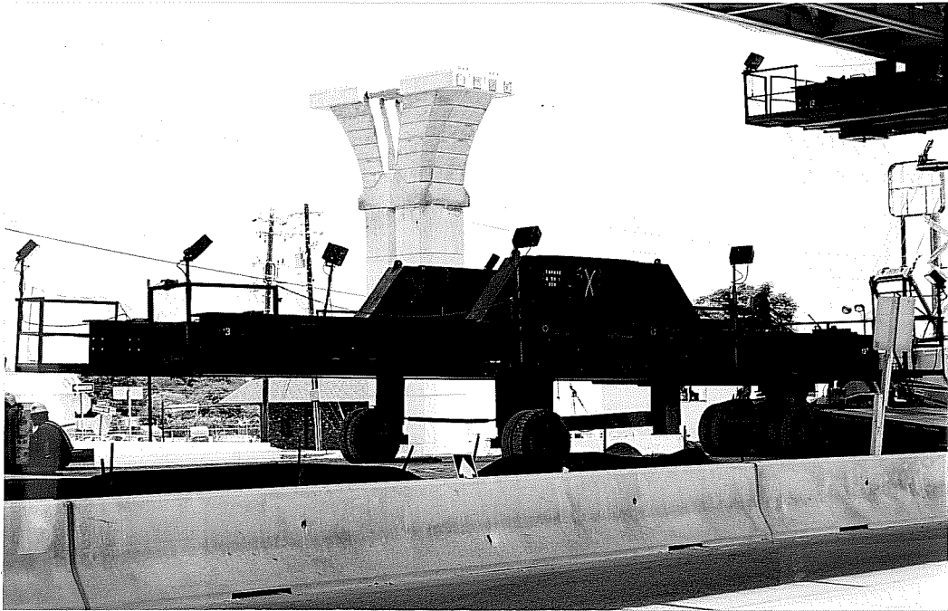
Figure 4.4 - Pier Bracket
