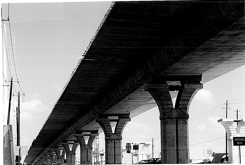
Figure 1. 2 - Photograph of US 183 Viaduct
